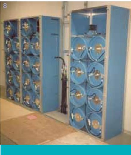
**Figure 8** Commercial use of beer barrel resonators at an airport. This system uses two antennas supplying ten and eight channels respectively
